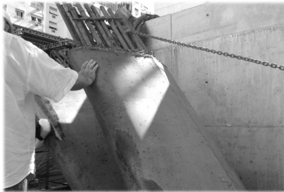
Prototype column: SCC, 50MPa, not vibrated
