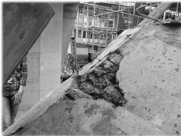
Prototype column: conventional concrete, usual procedures, 50MPa, slump 120mm, vibrated)
