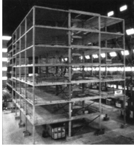
Cardington Concrete Building Frame
