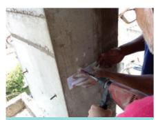
FOTO 7 - FUROS COM BROCA E FURADEIRA NO PILAR PARA COLETA DAS AMOSTRAS
