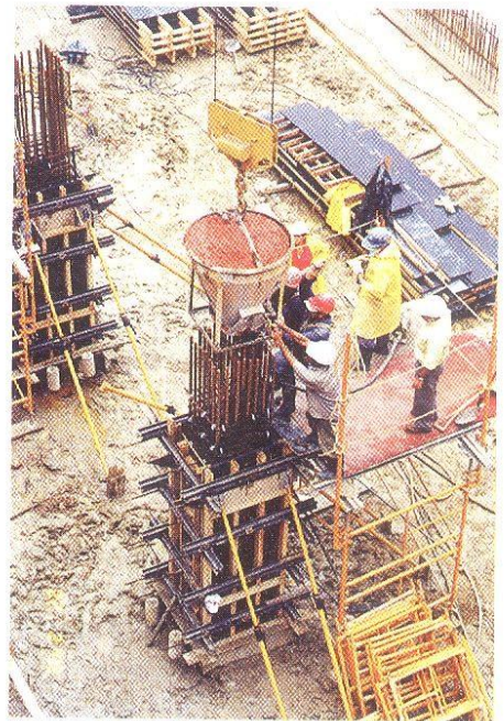
Fig. 5: A crane and dump bucket place HPCC into column formwork
