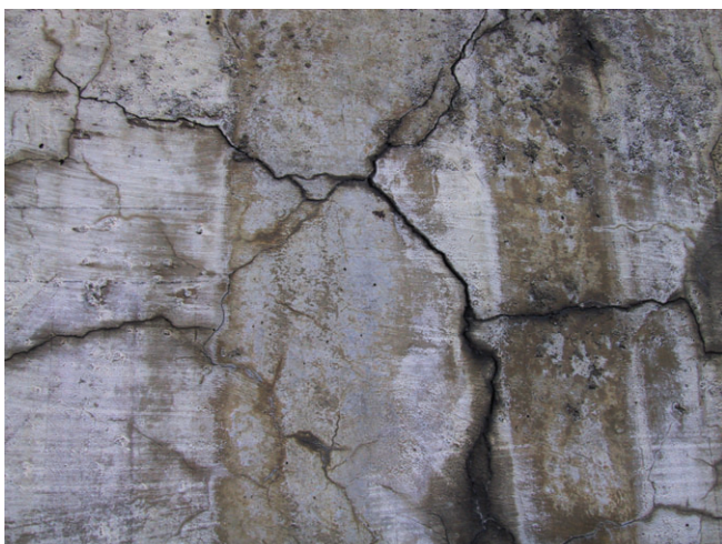
FIGURE 2 Leaching stains and map cracking (foundation block 7).
