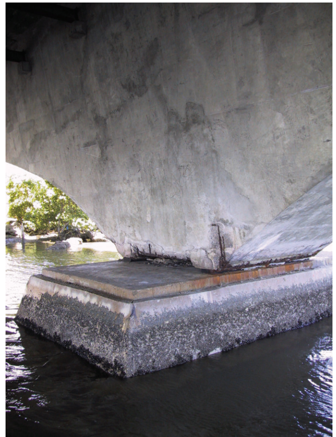
FIGURE 4 Severe steel corrosion on the superstructure of the Paulo Guerra Bridge.
