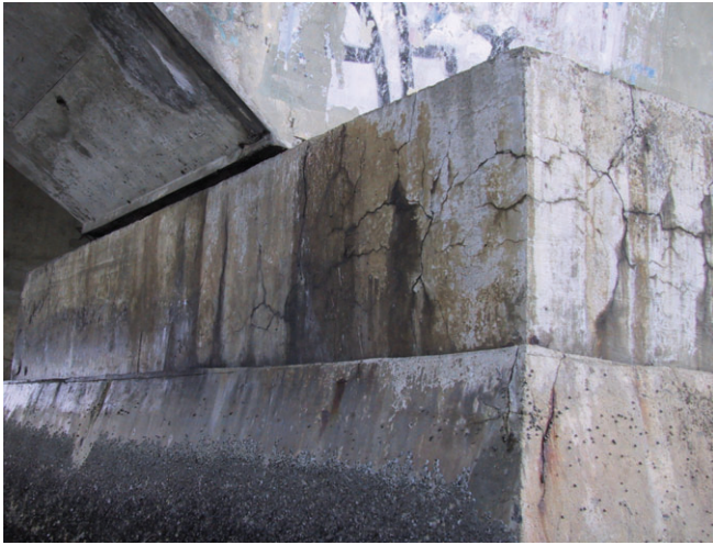
FIGURE 1 Signs of deterioration at the Paulo Guerra Bridge (foundation blocks, i.e., pile caps).
