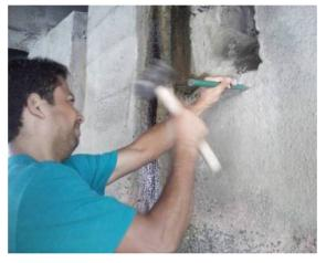
Figures 6: Breaking the surface of the concrete
