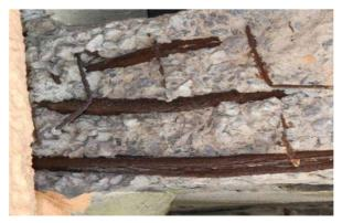
Figure 5: Beam section with disaggregation of the piece.
