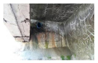
Figure 3: Cracks in beam of the Bridge.
