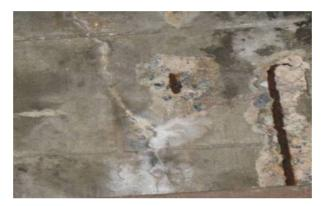
Figure 4: Fissures on the underside of the Bridge.
