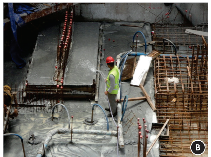
Figure 5 – Detail of concreted phase, joint to the reinforcing wall, with a curing mat over the surface and of curing procedure (mat being soaked)
