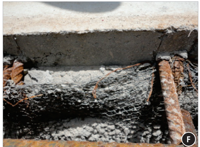
Detail of finishing obtained by upper wooden support barrier, wire mesh just underneath, will yet be cut
