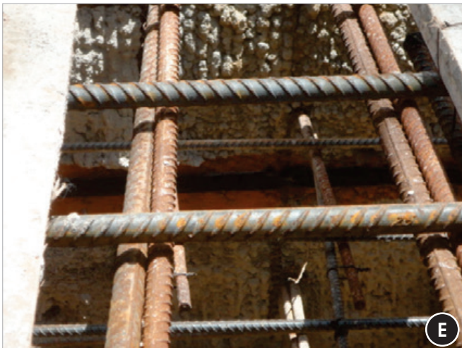
Detail of hydro swelling flexible tape already placed for next concreting procedure: reinforcement for next concreting phase is totally completed
