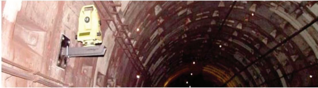
Figura 4: componente do ATMS ( AUTOMATIC TUNNEL MONITORING SYSTEM, 2011 ).
