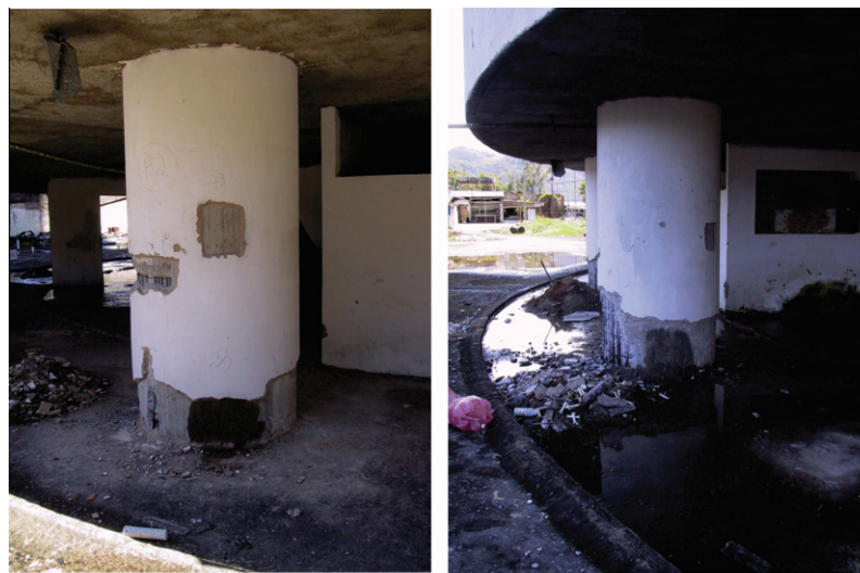
(a) P2 column, without water ponding. (b) P8 column, with water ponding.
