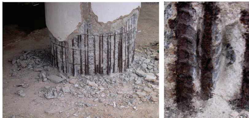
(a) corrosion at the column base at the ground level. (b) corrosion cell formed.
